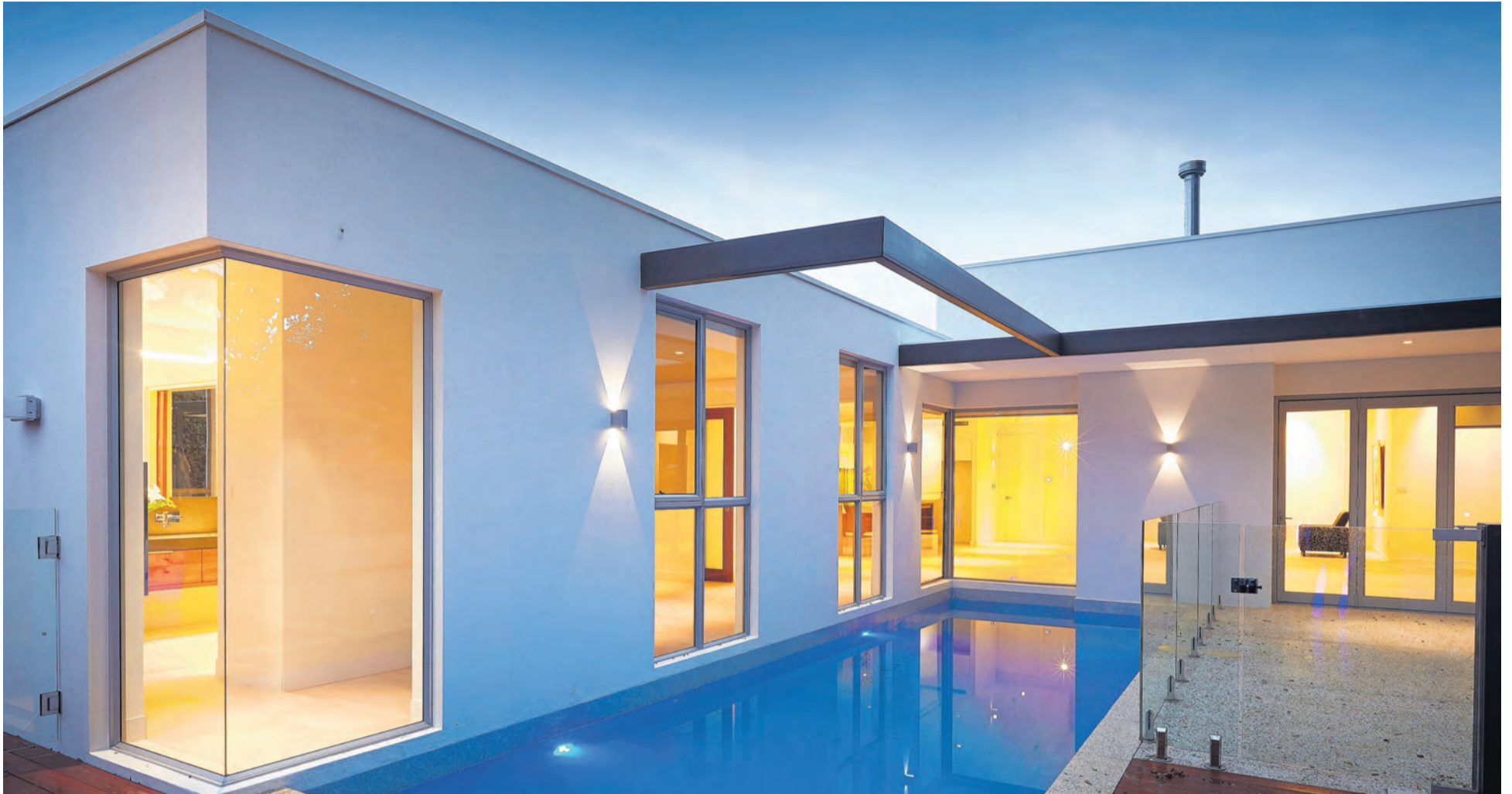
The 12m-long plunge pool can be seen from the living area and the main suite.
