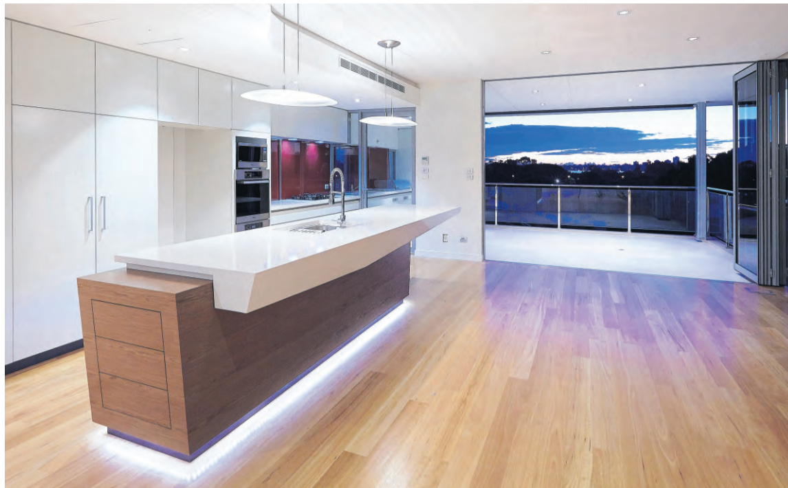
A 1.2m overhang meant the stonebench needed an individual, complicated design.
